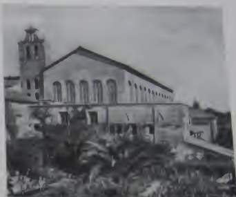
Fig. 68. S. Sabina. View from the east.
